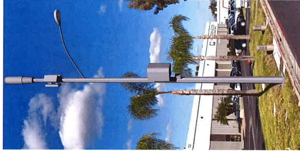
Street Light Pole VZW Typical Installations - #LS-AAL (Light Standard - Antennas Above Light)
